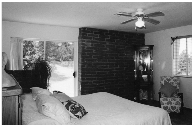
This is a solar wall built in a bedroom near a large sliding glass door. The bricks provide thermal mass to store the heat during the day and release it into the room at night.
